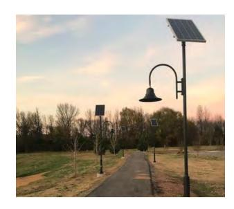
Figure 61. Solar powered lighting can be used along pathways without the need to connect to the electrical grid.
