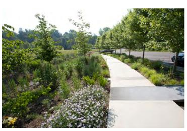
Figure 60. Bio-swales, similar to drainage ditches, utilize selected vegetation to filter and slow down stormwater runoff prior to its drainage into the water shed. These bio-swales can be designed using native vegetation adapted to the area, requiring minimal maintenance.
